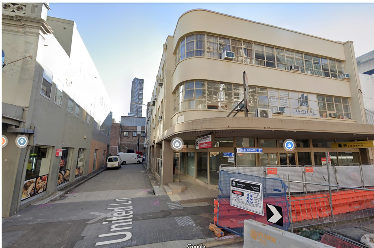
Figure 7-5: Street view of 48 Macquarie Street
