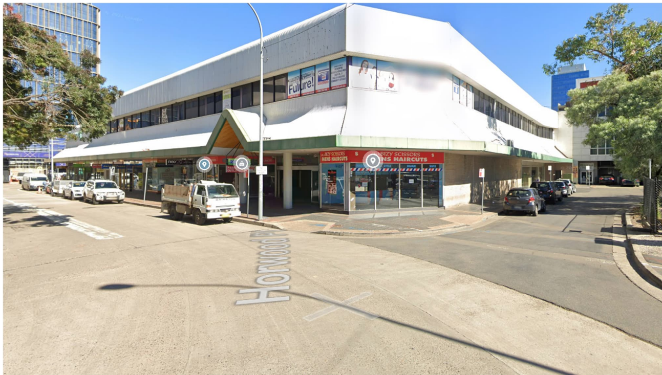
Figure 7-4: Horwood Place frontage
