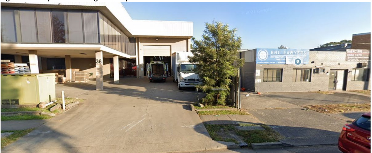
Figure 26: 36 and 38-40 Wentworth Street existing driveways
