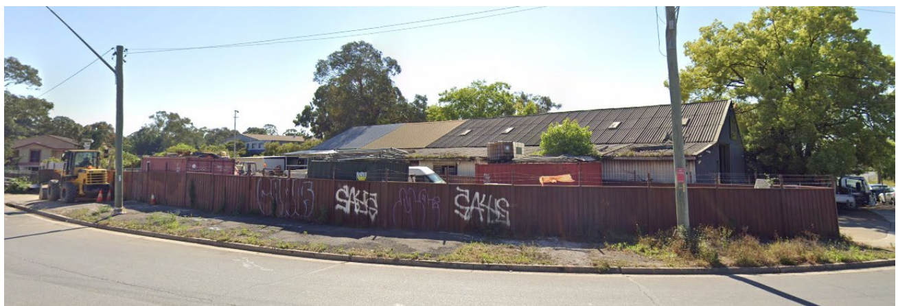
Figure 11: Kay Street/ Unwin Street footpath
