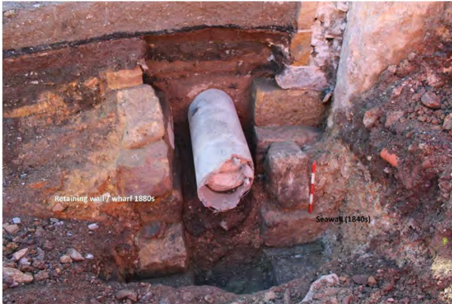
Plate 3: 1840s seawall and 1880s retaining wall uncovered at Balmain East, 2016
