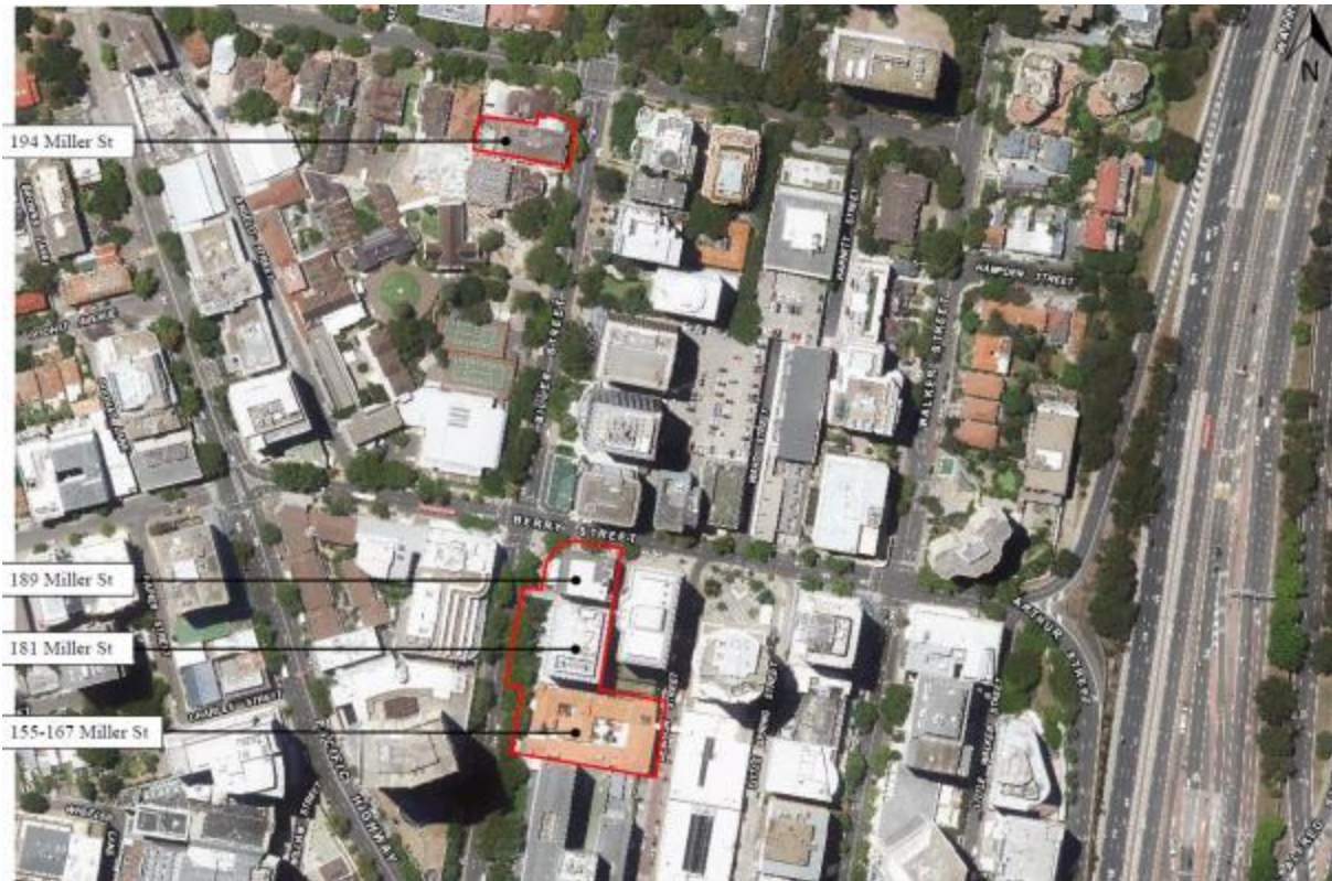
Figure 4 Demolition Sites VC1 and VC2
